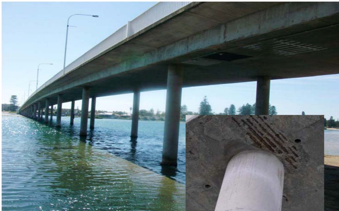
Figure 3-9 Bridge BC2 constructed in 1968 in Hunter region of NSW (Source: RTA)
