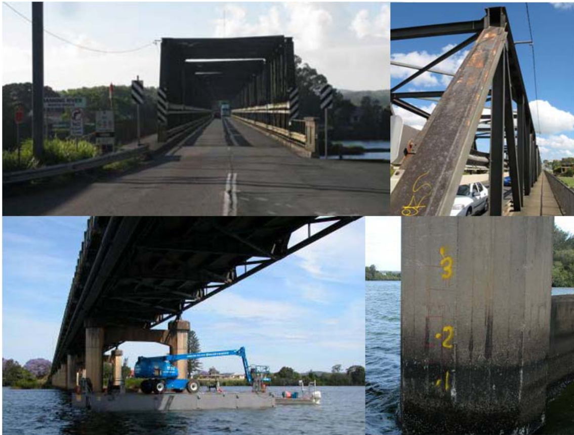
Figure 3-5 Bridge BC1 constructed in 1940, in Hunter region of NSW (Source: RTA)
