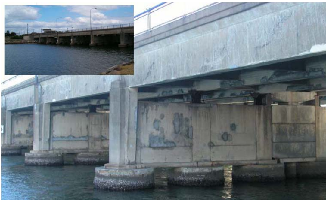
Figure 3-3 Bridge BB1 constructed in 1925 and 1959, in Sydney (Source: RTA)
