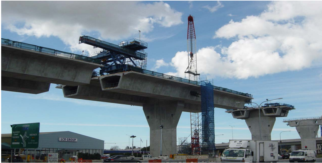
Bridge Construction (Source: CSIRO)
