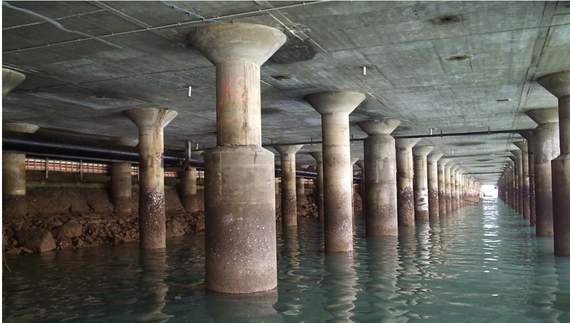
Strengthened concrete piles of port structures (SOURCE: CSIRO)
