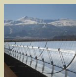
Andasol 1 and 2 Location: Spain Date of completion: Size: 50MW each Annual generation: 180GWh Source: Solar Millenium
