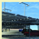
Menova Technologies, Canada Location: Ontario, Canada Date of completion: June 2008 Size: 28kW Source: Menova
