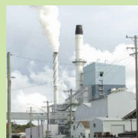
Earth Power technologies Location: Sydney Date of completion: 2003 Size: 3.5MWe Feedstock: Green waste and vegetable waste Source: Earth Power technologies
