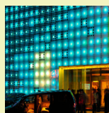
Jingya Greenpix Location: Beijing, China Date of completion: June 2008 Size: 79kW (2,200m 2 ) generating over 50MWh p.a. Capital cost: Integrated into façade costs. N/A Source: Arup project case studies
