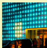
Jingya Greenpix Location: Beijing, China Date of completion: June 2008 Size: 79kW (2,200m 2 ) generating over 50MWh p.a. Capital cost: Integrated into façade costs. N/A Source: Arup project case studies
