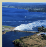
Annapolis Royal tidal plant Location: Bay of Fundy, Canada Date of completion: 1984 Size: 18 MW Annual generation: 50 GWh Source: Nova Scotia Power
