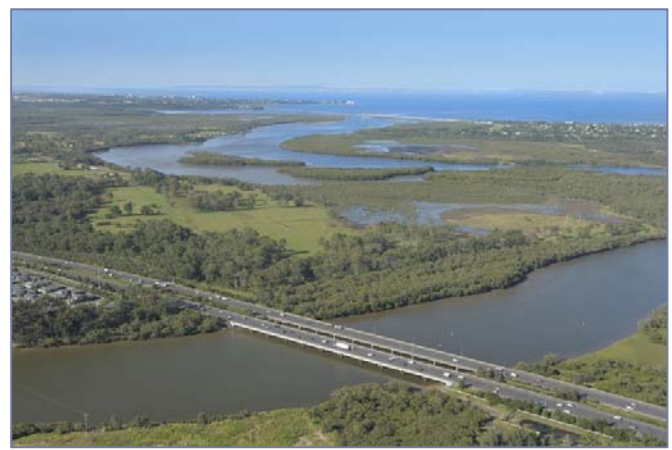
Figure 6 – Pine River Bridge (Source: MBRC)
