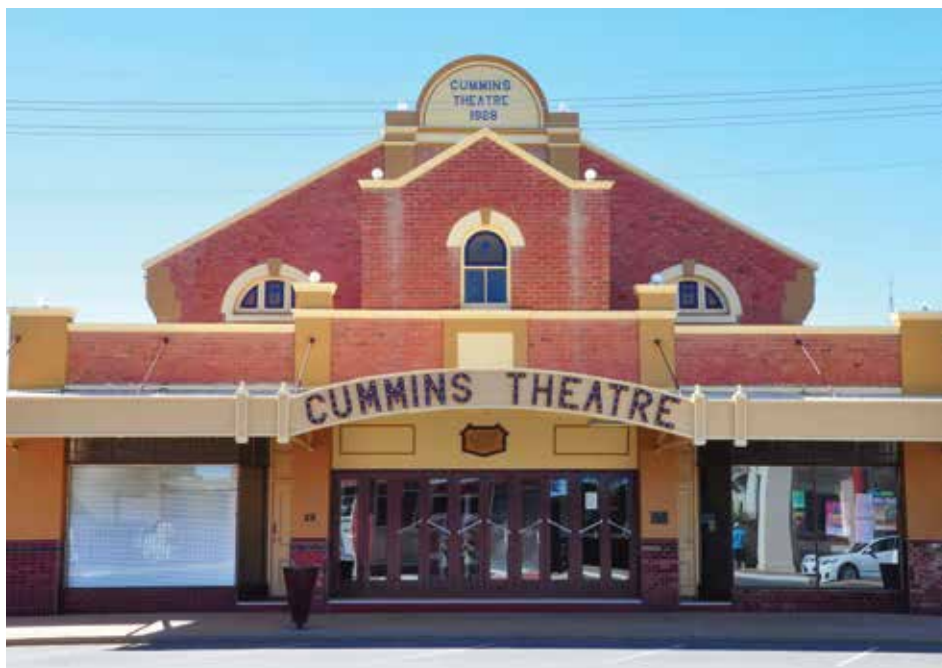
Cummins Theatre Conservation Works – Merredin Photograph courtesy of Chris Morris
