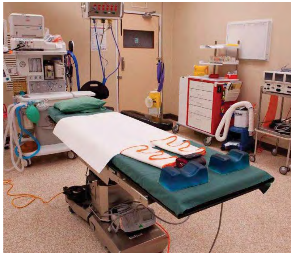
Nickol Bay Hospital operation theatre (Source DRD)
