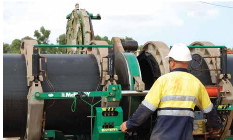
Gascoyne Irrigation Pipeline (Source DRD)
