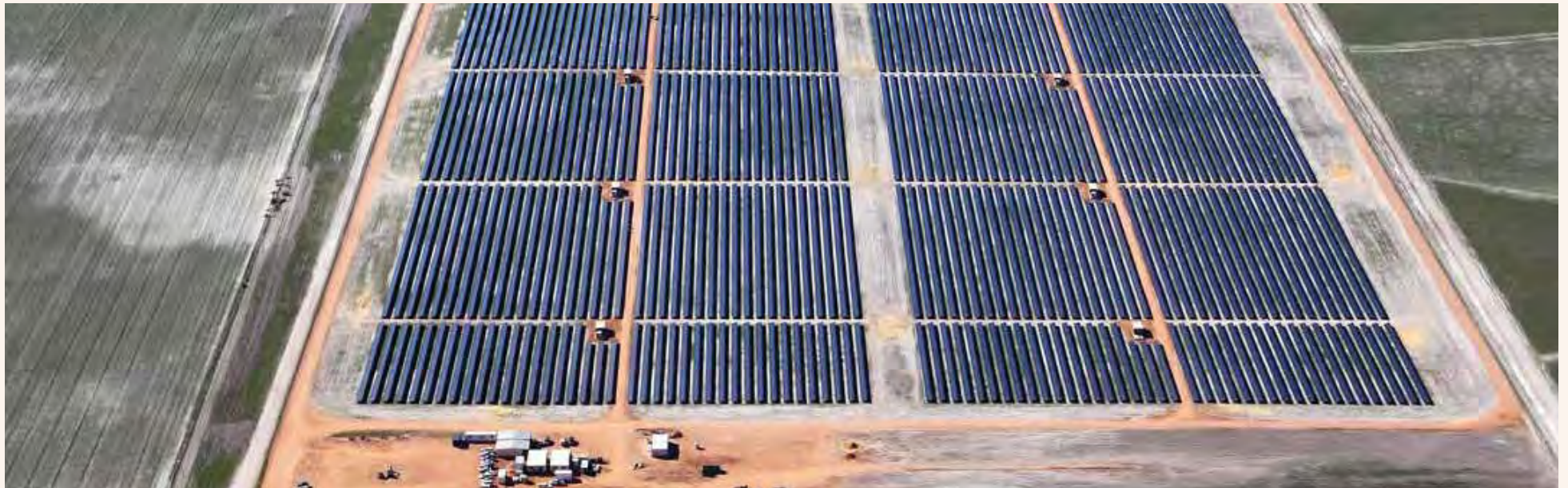
Aerial View of Solar Panels – Greenough River Solar Farm (Source DRD)
