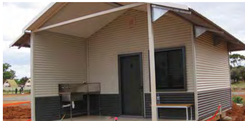
Kalgoorlie Indigenous Visitors Hostel Transportable (Source DRD)
