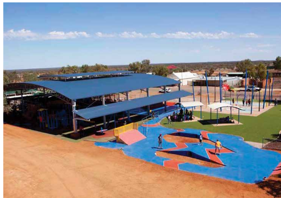
Yalgoo Community Hub – Covered Sports Facility (RageCage) Photograph courtesy of Rage Cage Sports Pty Ltd
