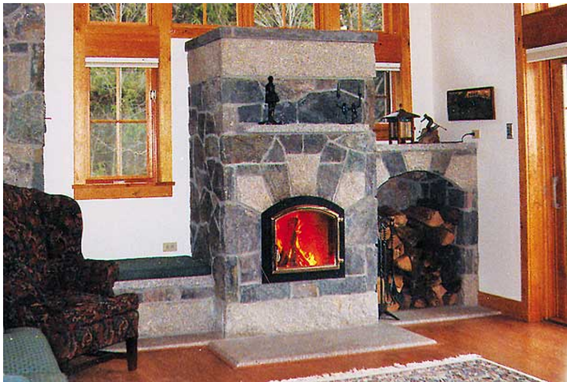
Figure 4.4 Example of a masonry heater.
