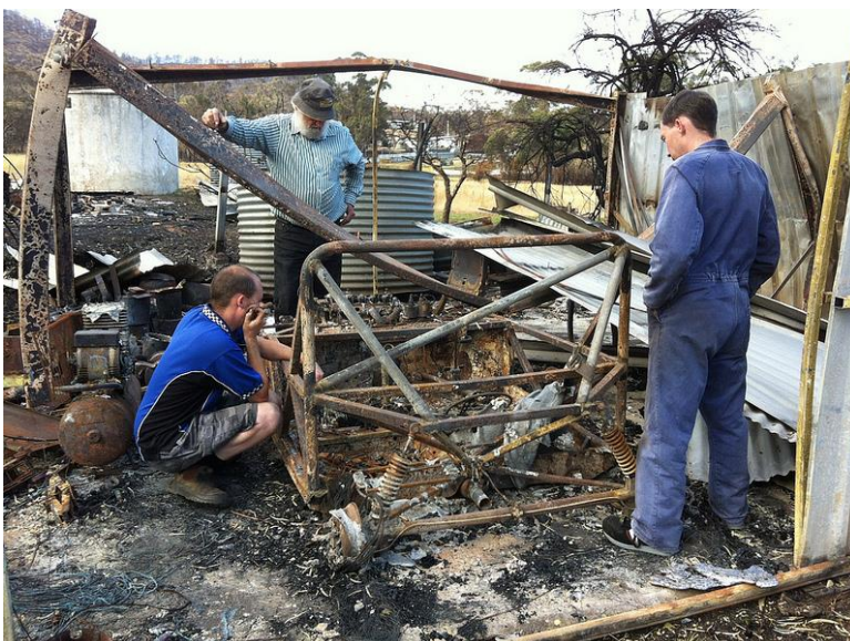
Photo 12. The 2013 bushfires highlighted the potential impacts of climate-related events on infrastructure. Photo: Sarah Brabazon
