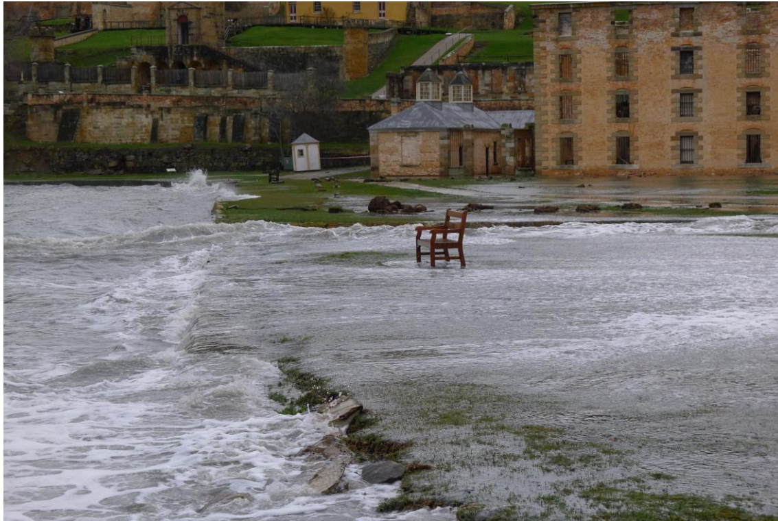
Photo 13. Storm damage to world heritage listed Port Arthur Historic Site, 2011, Photo: Port Arthur Historic Site Management Authority
