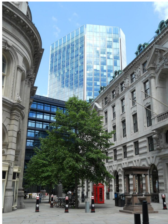
The London Stock Exchange, with its irregular façades, can be seen in the background. The entire building has been re-clad in glass.
