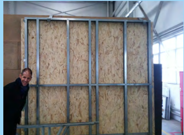
Figure 31 Case study 6 'flat pack' wall framing construction
