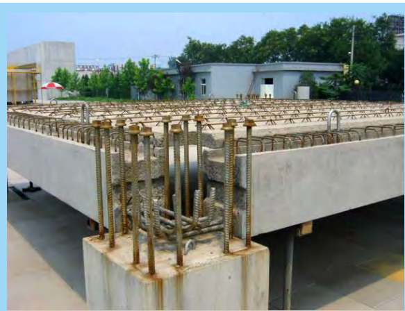
Figure 19 Prefabricated concrete structural products at case study factory yard
