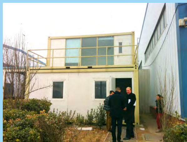
Figure 26 Case study 5 modular temporary office accommodation
