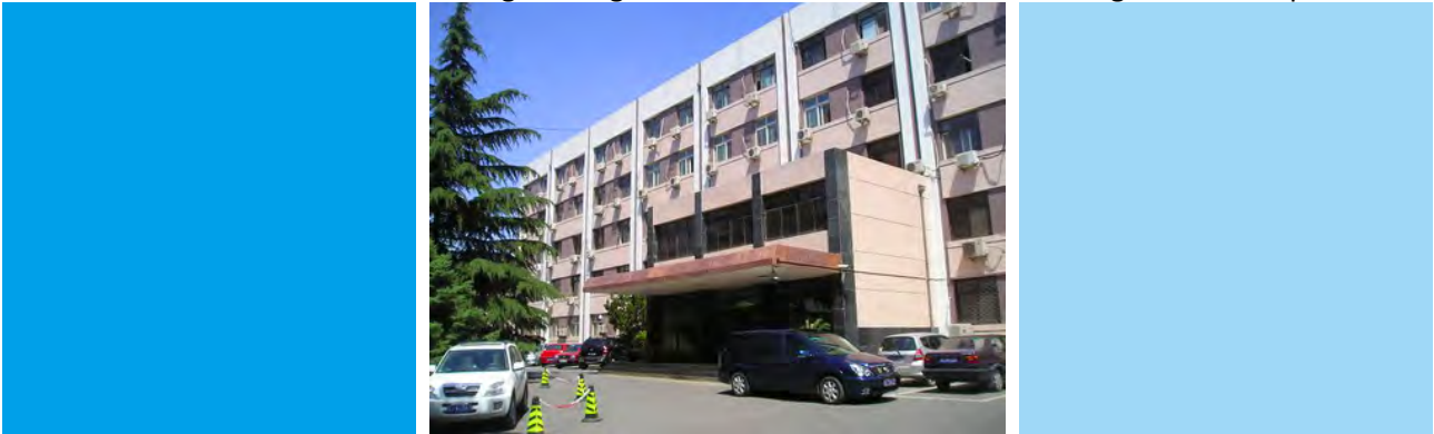
Figure 16 Headquarters Research Institute
