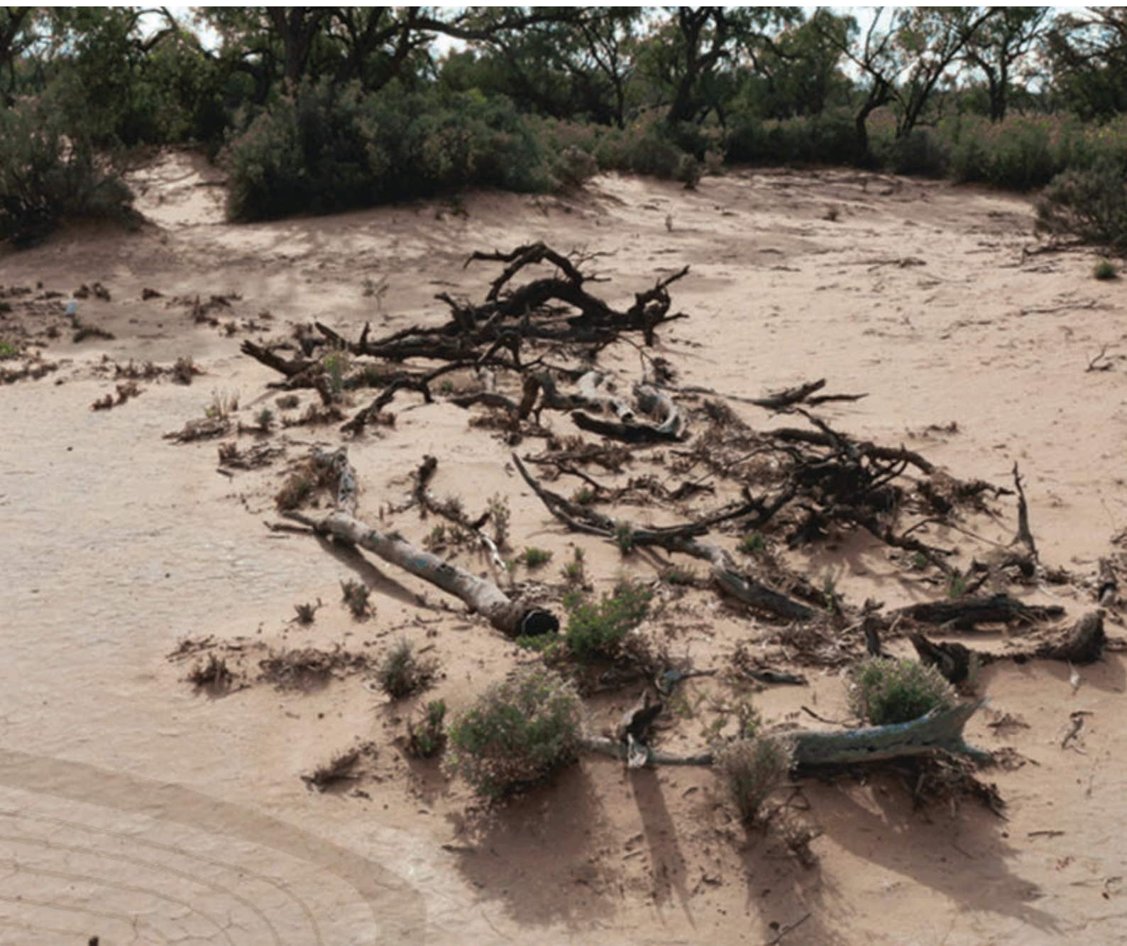
Burial protection works at Wallpolla Island. Photo by Darren Perry.
