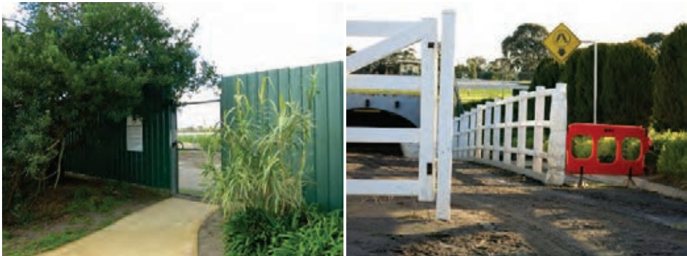
Neerim Road entrance—locked.
