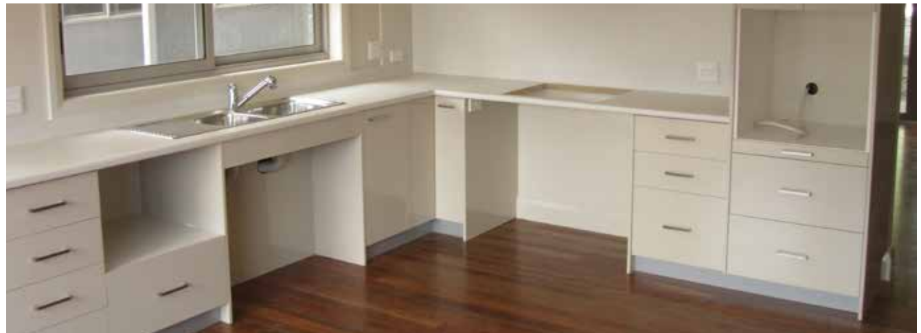
Underbench knee clearance and continuous flooring, kitchen, TAC RIPL housing.
