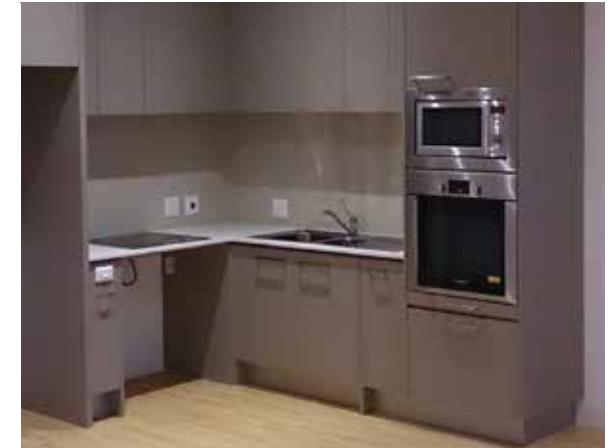
Removed underbench cabinetry post tenant modifications, Abbotsford
