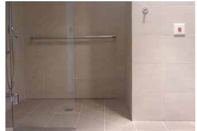
Ceiling-mounted 2-way speakers (above) and wall-mounted emergency call buttons (below), Abbotsford.
