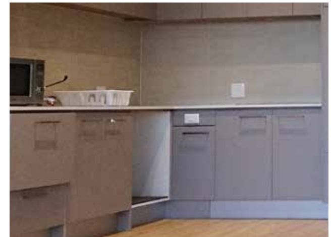
Post individual modifications, corner underbench cupboard removed to allow use of the cooktop by a person with reclined posture.
