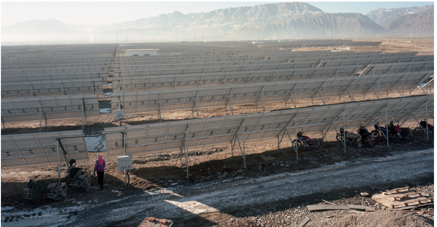
A solar farm under construction in the remote Gansu province, China.
