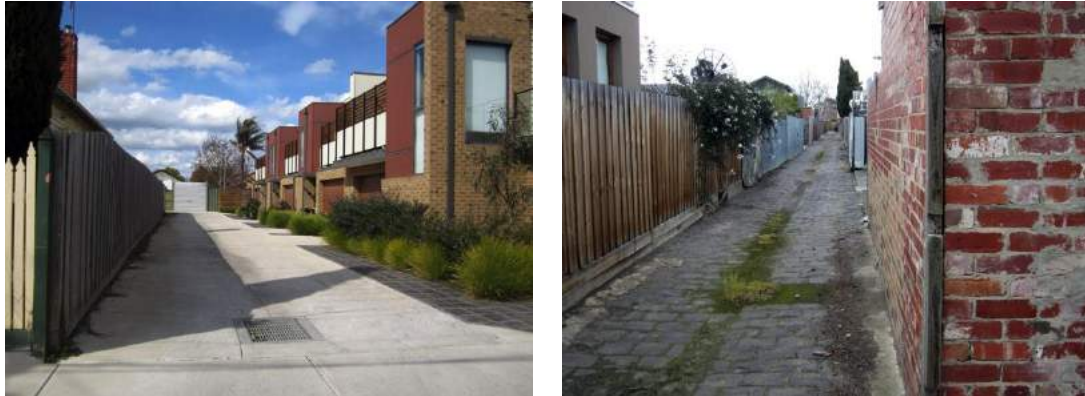
Figure 5. Townhouses and single family homes
