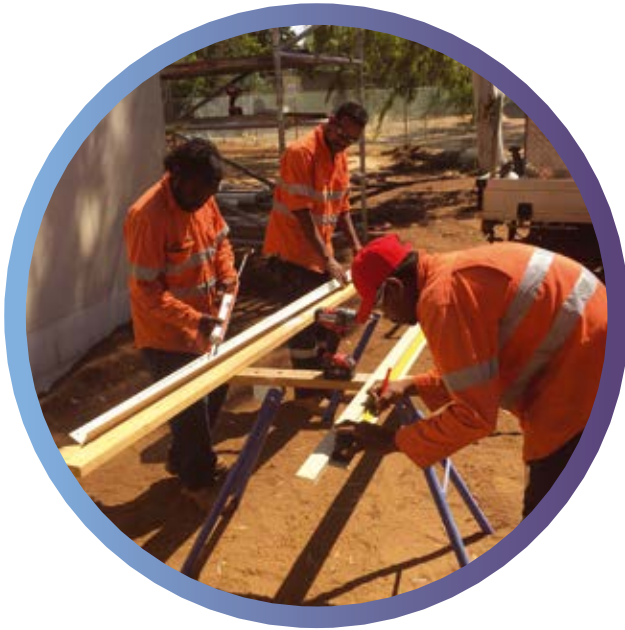
Jilkminggan community members (left to right) Stuart Yunupingu, Harry Albert and Matthew Conway at work building the community's new store.
