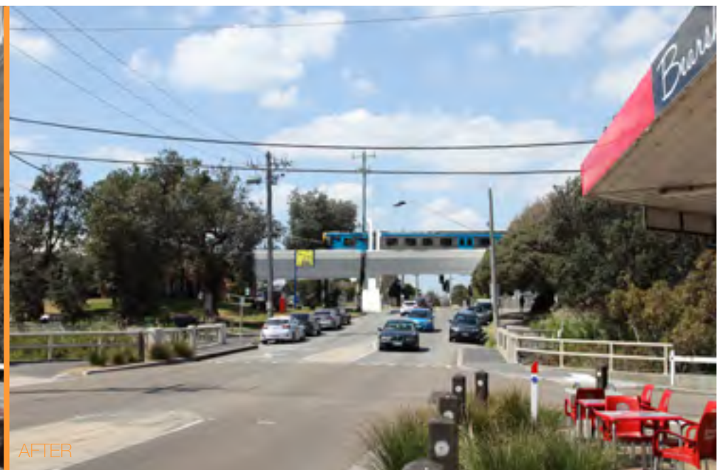
BELOW: Level crossing removal using elevated rail at Seaford - Chris Marinopoulos
