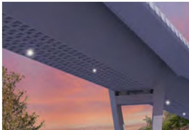
Concrete with soffit coffering pattern- Vincenzo Armenia
