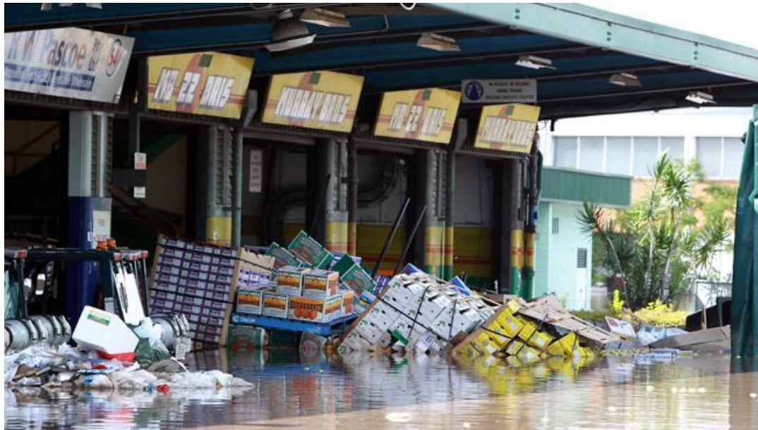
Above: The January 2011 floods devastated Brisbane's biggest fresh fruit and vegetable market at Rocklea. The 77-hectare site was completely inundated with flood water, resulting in a $100 million damage bill. Photo: Glenn Hampson
