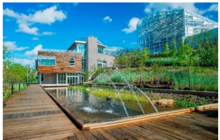
Figure 2. Phipps Center for Sustainable Landscapes, in Pittsburgh, Pennsylvania, used green infrastructure as one of its strategies to achieve SITES and LEED certifications.
