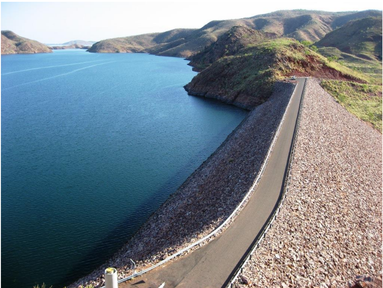
Figure 1: Ord River Dam Wall. Source: Nullysontheroad, Flickr
