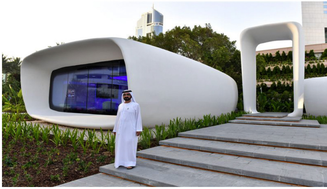
Fig. 3. Office building in Dubai printed by WinSun.
