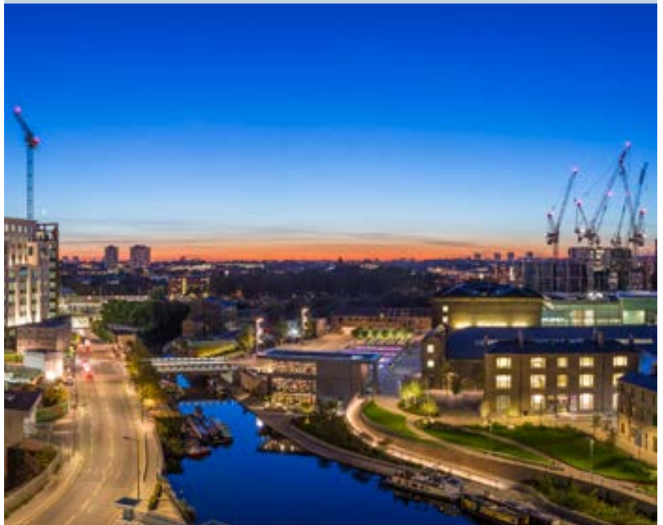
The buildings of Pancras Square, Waitrose and Arthouse at the King's Cross redevelopment project in London
