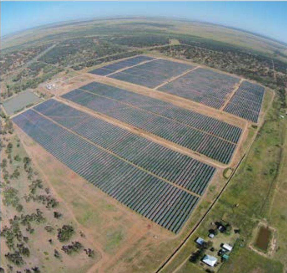
Foresight Group's 25MW solar farm at Barcaldine, Queensland
