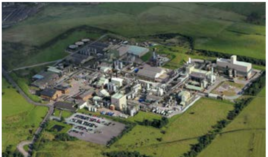
Nufarm's manufacturing facility in Wyke
