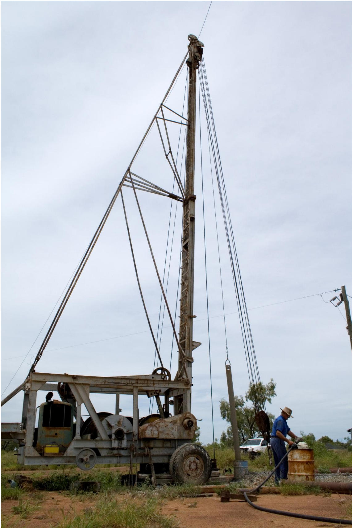
WORKING BORE RIG. PHOTO: GABCC
