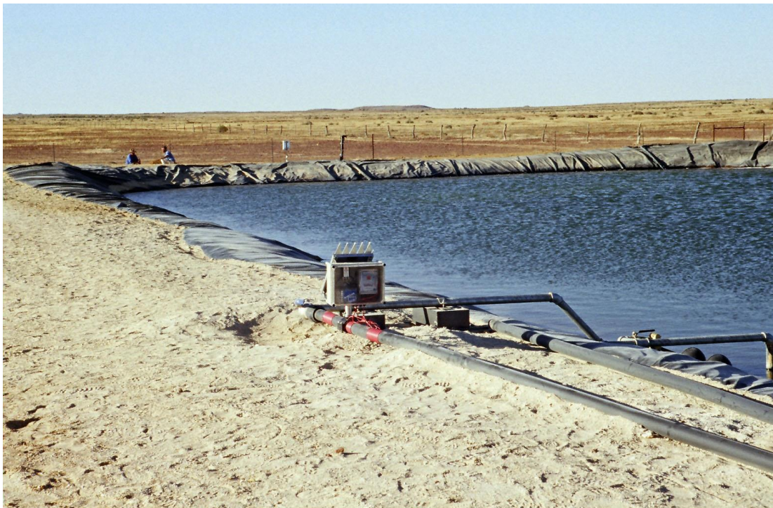
COOLING POND FOR ARTESIAN WATER, BIRDSVILLE TRACK, SOUTH AUSTRALIA, 2002. PHOTO: G HOGAN
