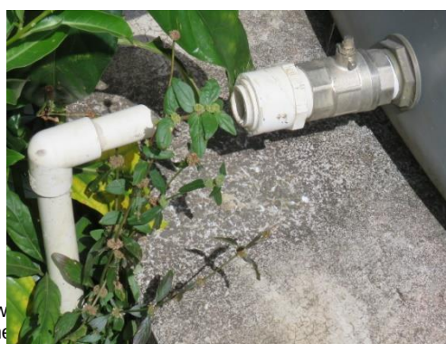
Figure 2 Vaivase Primary School broken pipe from water tank
