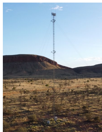
Figure 4: Warakurna mobile tower
