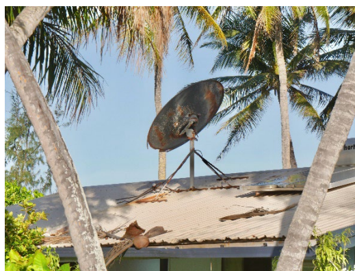
Figure 19: The proximity to salt water in Erub causes rapid corrosion of satellite dishes
