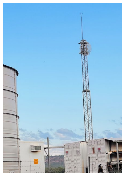
Figure 13: The HCRC repeater tower located at the water plant
