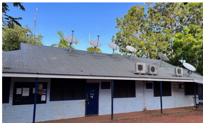
Figure 32: Four nbn Sky Muster dishes on the Kalumburu community office provide backhaul for the Wi-Fi mesh network
