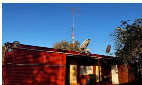
Figure 21: The CRC has been repurposed as a local enterprise printing facility, with one community access computer
