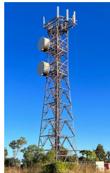
Figure 5: The Galiwin'ku mobile tower with microwave repeater links from the mainland
