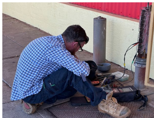
Figure 22: Technician doing maintenance on the Telstra fixed line network
