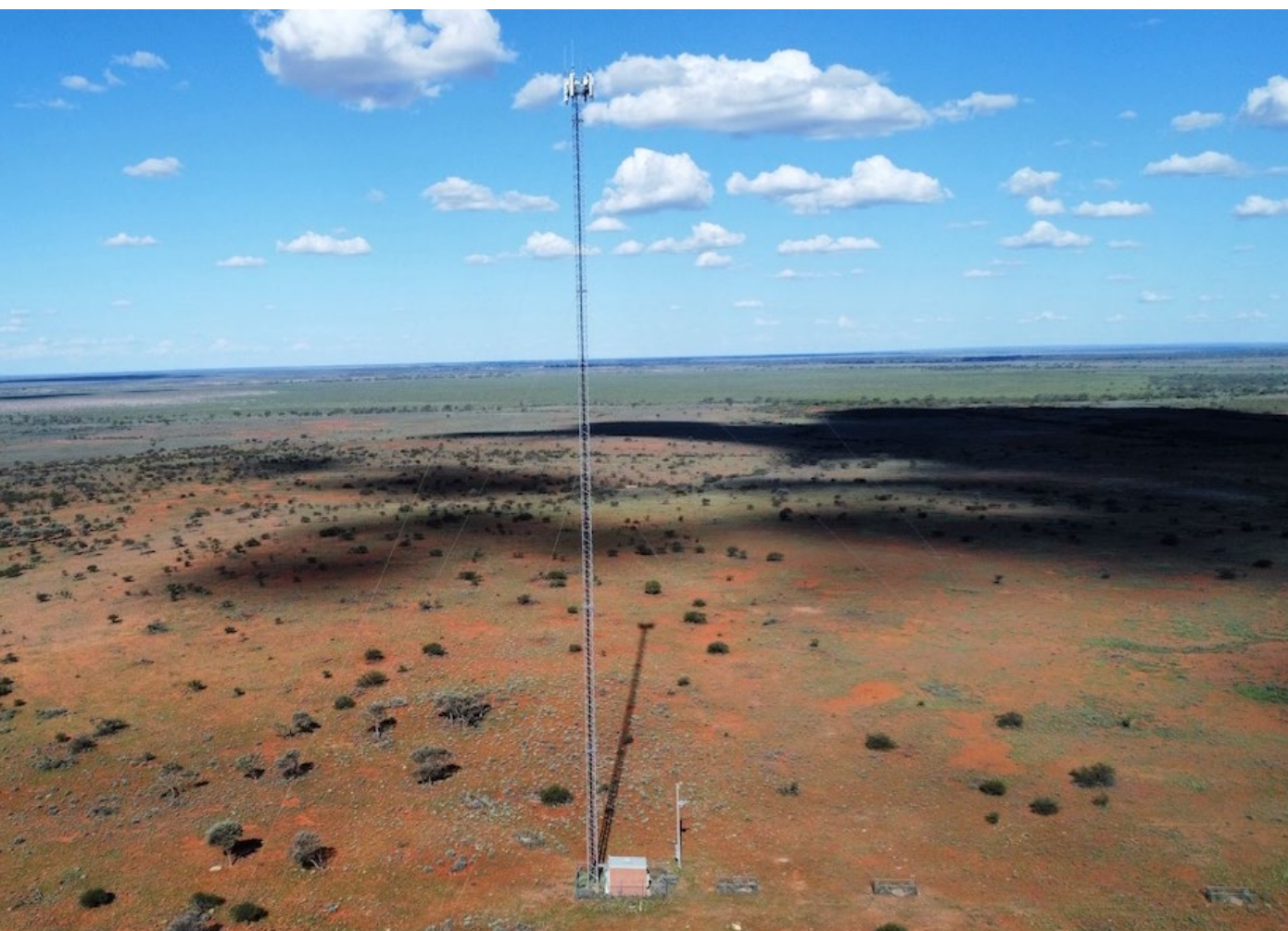
Figure 8: Telstra 4G/5G Mobile tower at Netallie Trig, 11km west of Wilcannia
