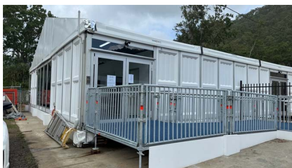
Figure 22: The newly opened temporary Wujal Wujal clinic, May 2024
