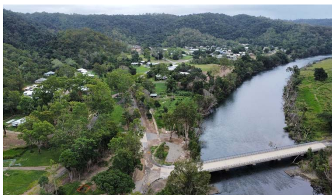
Figure 19: The western side of town (in bottom half of photo) and foothills (right of bridge) are in a signal shadow zone from the Mt Pearce mobile tower
