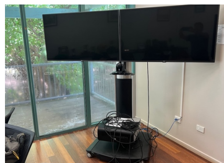
Figure 20: Videoconference facility in TSIRC Boardroom
