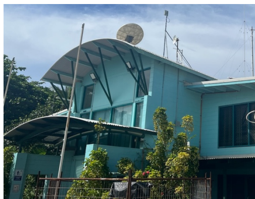
Figure 17: TSIRC building with NBN Sky Muster dish and Wi-Fi access point on roof
