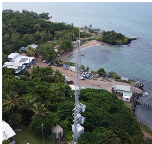
Figure 9: Telstra mobile tower in Medige Village
