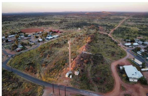
Figure 2: Aerial photo showing the new 4G tower on the ridge in the centre of Yuelamu
