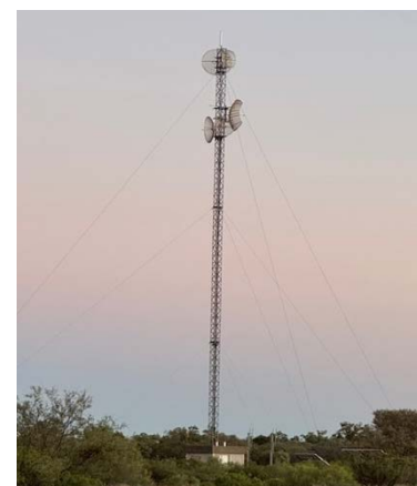
Figure 6: Telephony was delivered to Yuelamu via a regional HCRC microwave repeater network
