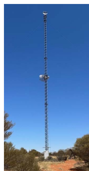
Figure 7: HCRC repeater tower
