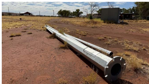
Figure 12: Sections of the small cell mobile tower awaiting construction in Kalka
