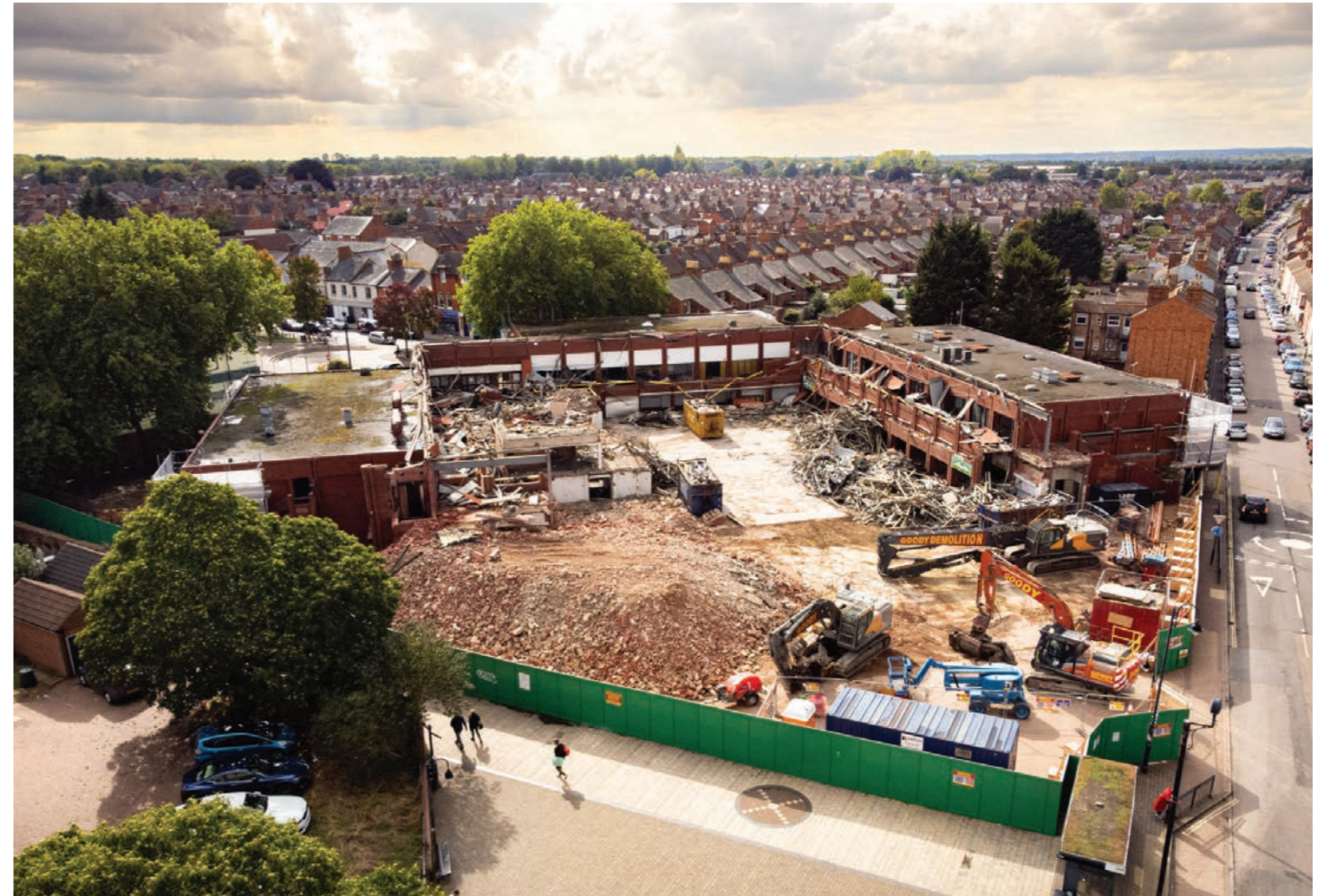
Figure 16: The Agora's demolition site in 2022 Source: https://lovewolverton.co.uk/demolition-update/
