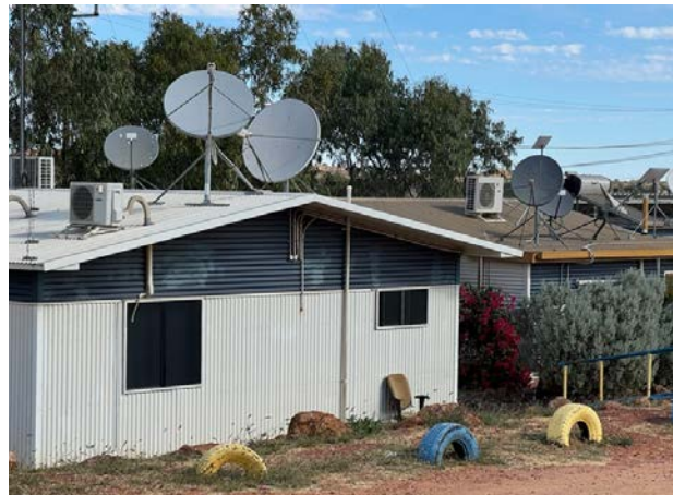
Satellite dishes on Central Desert Regional Council office, Yuelamu
