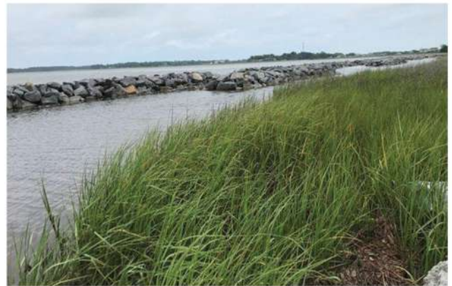
Granite rock sill in combination with salt marsh revegetation (Swansboro, North Carolina, US)
