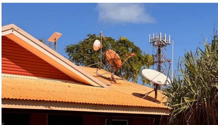
Figure 8: A Starlink dish (left) among an array of communications equipment on the East Arnhem Regional Council office
