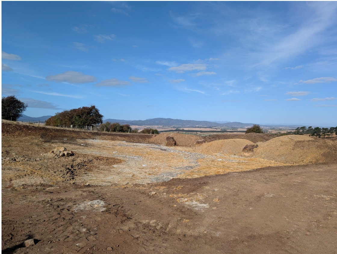
Figure 1.3 Exposed bedrock after contaminated soil was removed from part of the site
